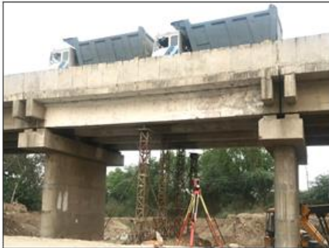
Fig 1: - Bridge Load Testing
